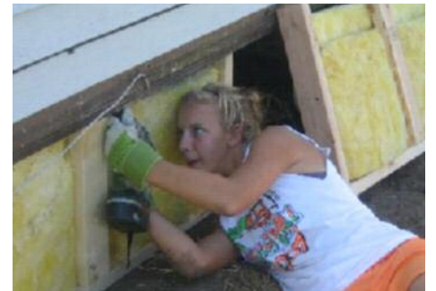
Kenzie Kennedy toe-nailing skirting to a trailer home.
